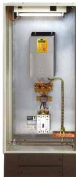
DC590+ DRV equivalent illustrating panel space saving
